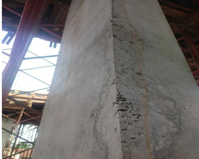
Figure 1. Delamination In A Column
