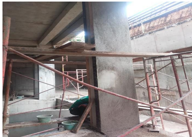
Figure 2. Repair Process Using The Plastering Method
