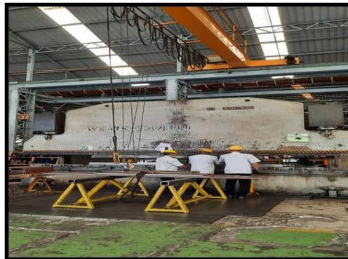
Figure 11. Bending process on bottom flange
