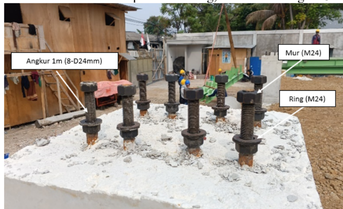
Figure 3. Embedded Anchors in Concrete Columns
