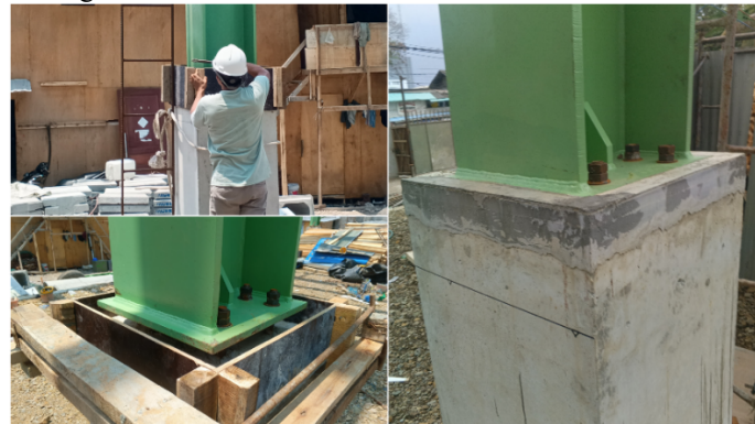
Figure 5. Grouting Work Process
