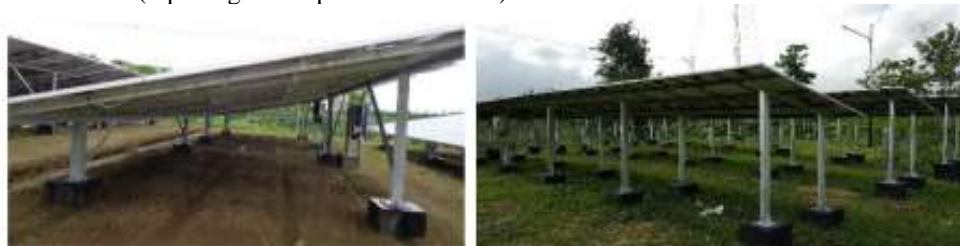
Gambar 1. Contoh Jenis PLTS Ground Mounted
