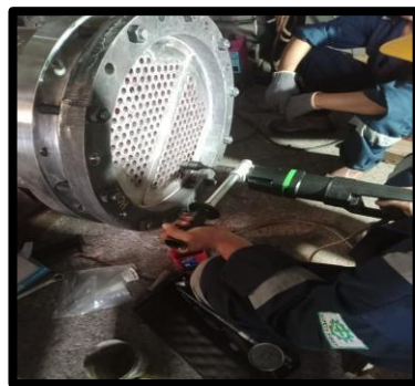
Gambar 9. Proses Expand
