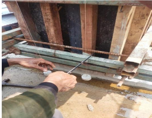
Figure 11. Column Verticality Inspection Using Plumb Bobs
