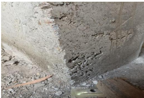
Figure 9. Porous Column
