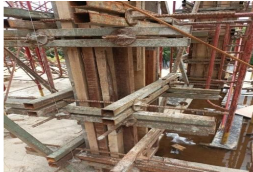
Figure 4. Column formwork
