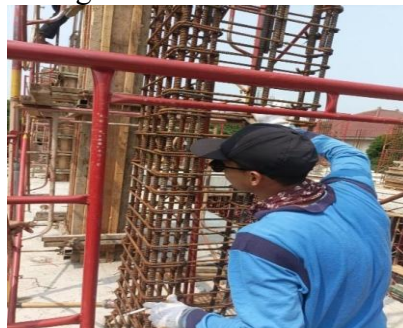
Figure 1. Column reinforcement
