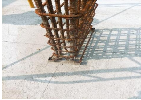
Figure 2. Installation job of column shoes
