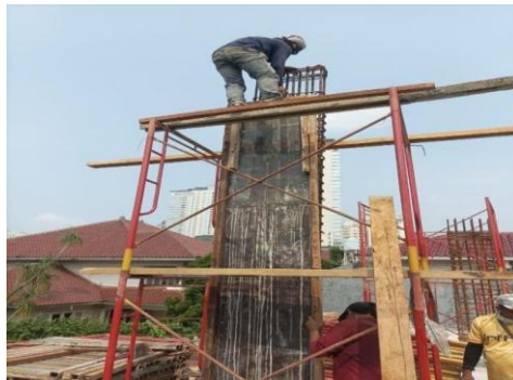
Figure 3. Formwork installation
