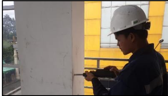
Gambar 9. Proses Pengujian Hammer Test
