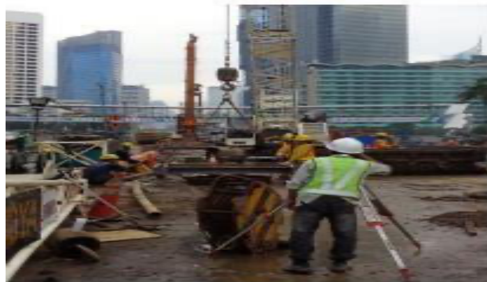
Figure 11. Installation of the king post table
