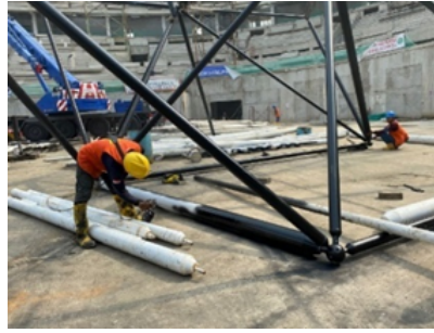
Figure 5. Space Frame Module Painting Process
