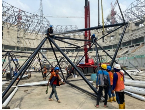
Figure 7. Space Frame Module Assembly
