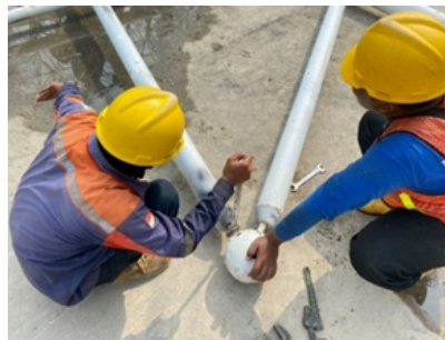
Figure 4. Space Frame Module Assembly Process
