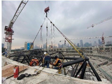
Figure 9. Space Frame Module Erection Process
