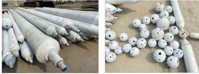
Figure 3. Space Frame Material Sorting Process
