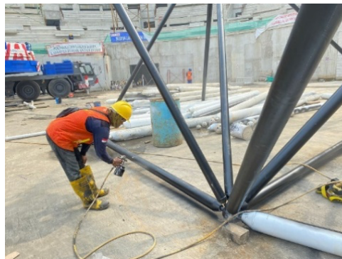
Figure 8. Space Frame Module Painting
