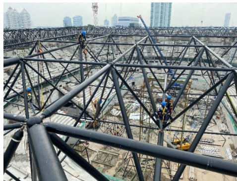
Figure 10. Space Frame Module Merging Process for Each Zone
