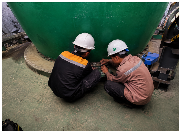
Figure 2. Electrical Inspection Activities at PT Dean Shoes
