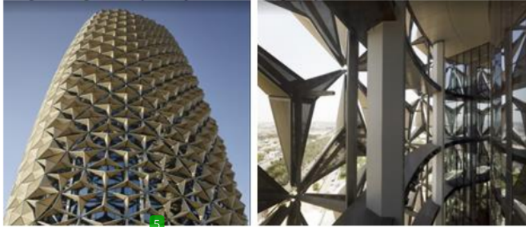
Gambar 5. Kinetic Facade di Abu Dhabi Investment Council New Headquarters - Al Bahr Towers Sumber: https://archello.com/story/36573/attachments/photos-videos/6 (2023)
